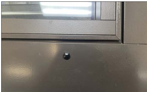
NYLON PLASTIC SNAP-IN PLUG INSTALLED ON A BRONZE FINISH 8500 SERIES
