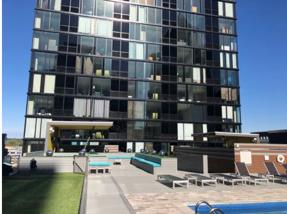
Custom Window Wall System with 1,161 Fixed Windows
