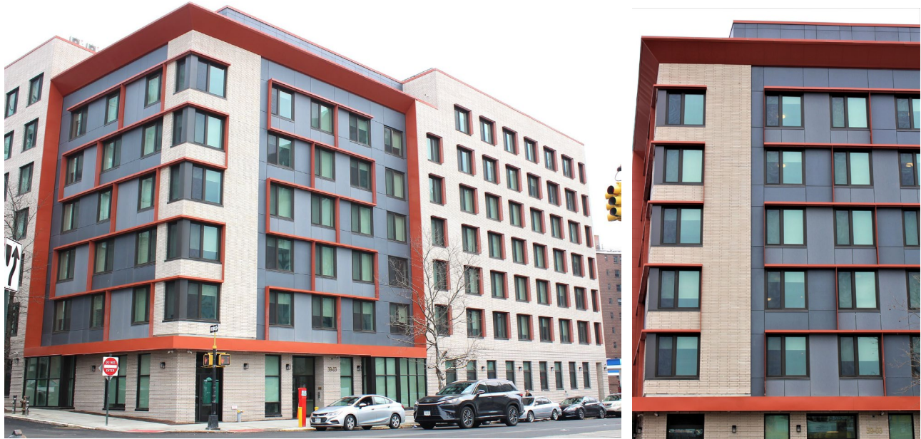
Crystal supplied commercial vinyl uPVC windows for newly constructed Magnolia Gardens in Flushing (Queens), NY, which provides transitional housing for families.
