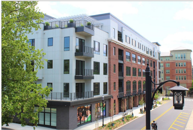
Crystal windows with narrow sightlines and great strength offer residents of The Mosaic abundant daylight, multiple styles and functions, and effective sound attenuation, important due to the proximity of the property to the South Orange NJ Transit rail station.
