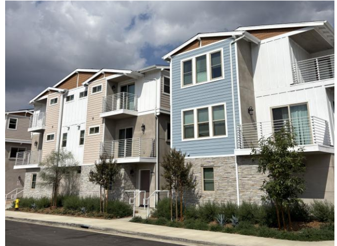
The new Crystal windows and doors at Heritage on First have extruded beige vinyl frames and many notable features.
