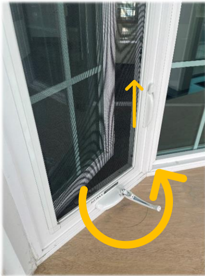
Open: Unlock the frame lock and turn the crank counterclockwise
