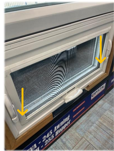
Lock the window by flipping the latches downward
