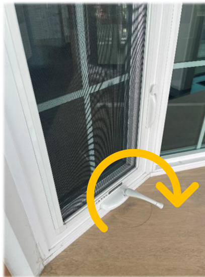
Close: Keep the lock unlocked and turn the crank clockwise
